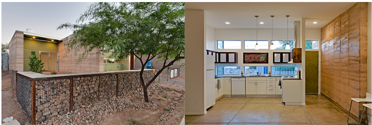
Figure 4: plit House; hybrid rammed earth thermal mass and insulative framed walls. (Photo: Liam Frederick)
